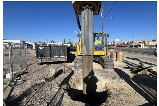
Drilling for the new signal across from RSIC
